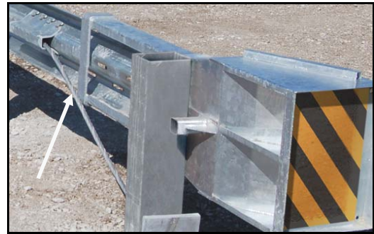
FLEAT-SP-MGS cable NOT to be fed inside the feeder chute
