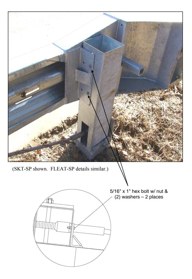
Figure 10. Impact Head Connection Detail for <u>SKT-SP</u> & <u>FLEAT-SP</u>
