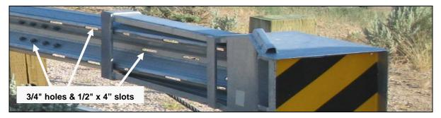
The **SKT-SP** may use an end panel with only three (3) slots  $\frac{1}{2}$ " x 4" in the valley of the rail. The **FLEAT-SP** may use an end panel with only ten (10) slots  $\frac{1}{2}$ " x 4" in the corrugations of the rail. The other W-Beam railing sections in the **SKT-SP** or **FLEAT-SP** shall be the same used in highway guardrail with 6'-3"post spacing.
