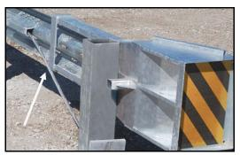
The **SKT-SP** cable is fed inside through the feeder chute. The SKT feeder chute is longer than the FLEAT
