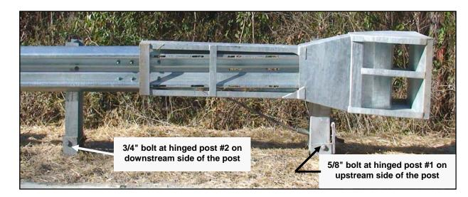
Figure 6. Post #1 Connection Detail for <u>SKT-SP</u> & <u>FLEAT-SP</u>
