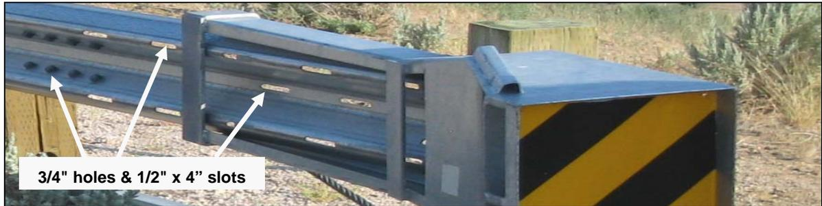
The **SKT-SP** may use an end panel with only three (3) slots  $\frac{1}{2}$ " x 4" in the valley of the rail. The **FLEAT-SP** may use an end panel with only ten (10) slots  $\frac{1}{2}$ " x 4" in the corrugations of the rail. The other W-Beam railing sections in the **SKT-SP** or **FLEAT-SP** shall be the same used in highway guardrail with 6'-3" post spacing.
