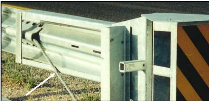
The **SKT-SP** cable is fed inside through the feeder chute.
