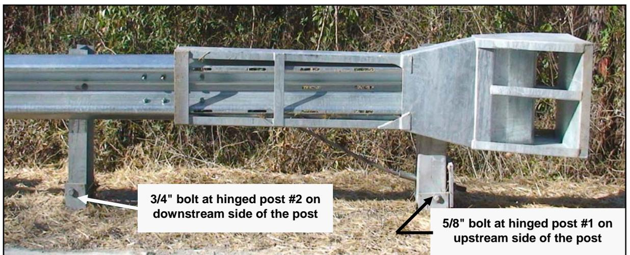
**Figure 6. Post #1 Connection Detail for SKT-SP & FLEAT-SP**
