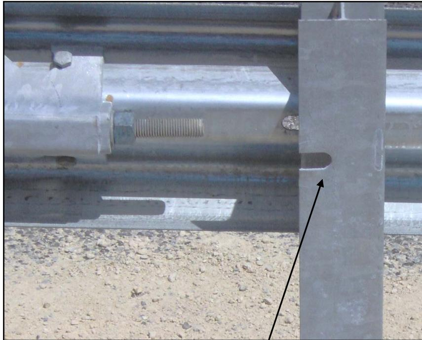
There is an open-ended slot in the flange of the post at the post bolt connection. Be sure upper post #2 is installed with this slot facing post #1.
