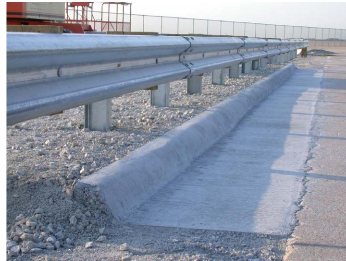
FIGURE 3 Midwest Guardrail System for Special Applications: (a) Quarter-Post Spacing (Design B), (b) Standard Post Spacing With AASHTO Type B Curb (Design C) [1 in. = 25.4 mm].
