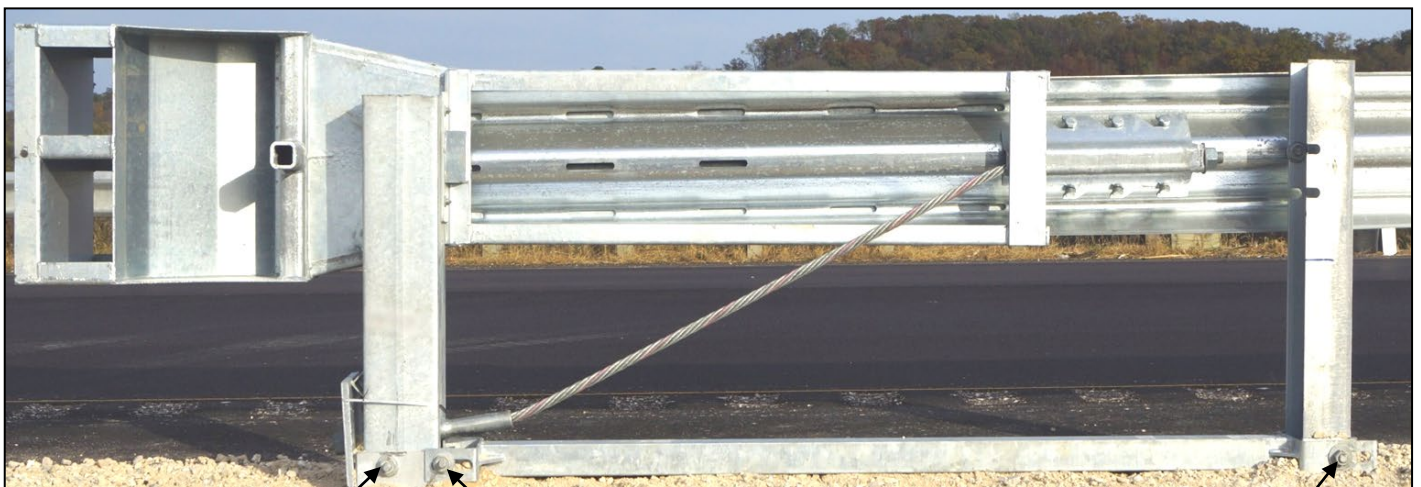
Post #1 Connection Detail
