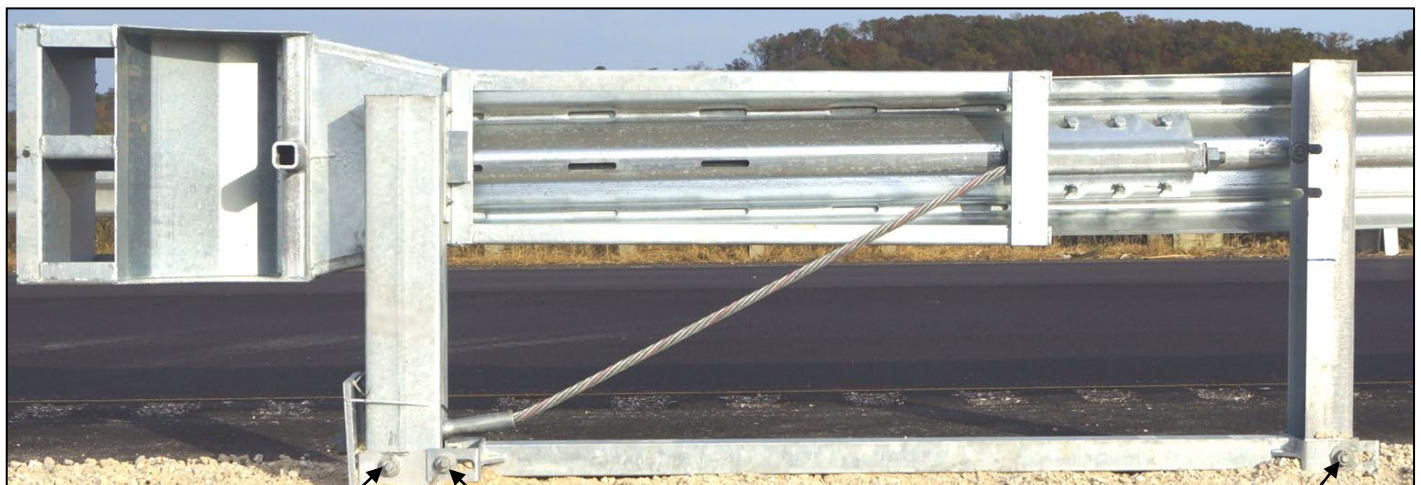
Post #1 Connection Detail
