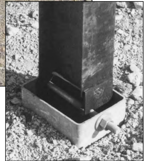
Plug Welded Steel Posts – In Foundation Tube
