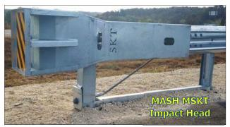
The MSKT Impact Head is able to be used on NCHRP 350 SKT units for new installations or for repairs. **ADDING THE MSKT IMPACT HEAD DOES NOT RETROFIT NCHRP 350 SKT INTO THE MSKT**. The letters "SKT" are cut into the traffic side of the MSKT Impact Head. This is because there will be NCHRP 350 SKT installations and there will be MASH MSKT installations, both with the same head. The other changes noted above will distinguish the MASH MSKT from the NCHRP 350 SKT.
